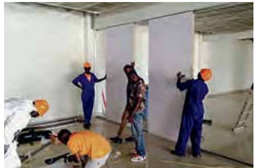
Installation of STRAWTEC laminated partitions
