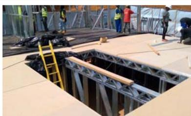
*STRAWTEC Slab being fitted to a metal frame, Kigali*
